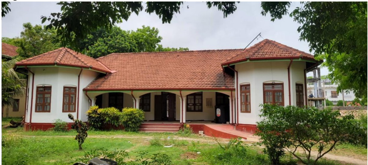
Rogers Home After refurbishment
