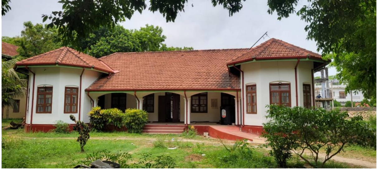
Rogers Home After refurbishment
