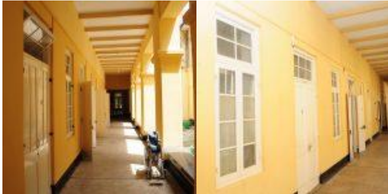
Jameson Block after repairs
